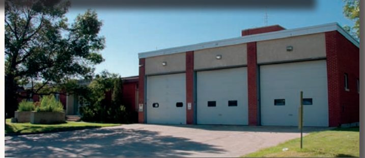
Before renovation when the building was still the police station and fire hall
