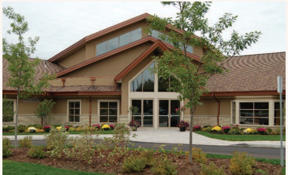
Close up of the main entrance
