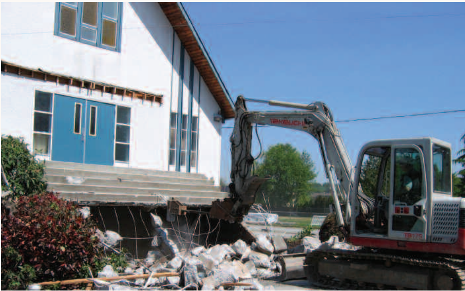
Bulldozing the front steps.
