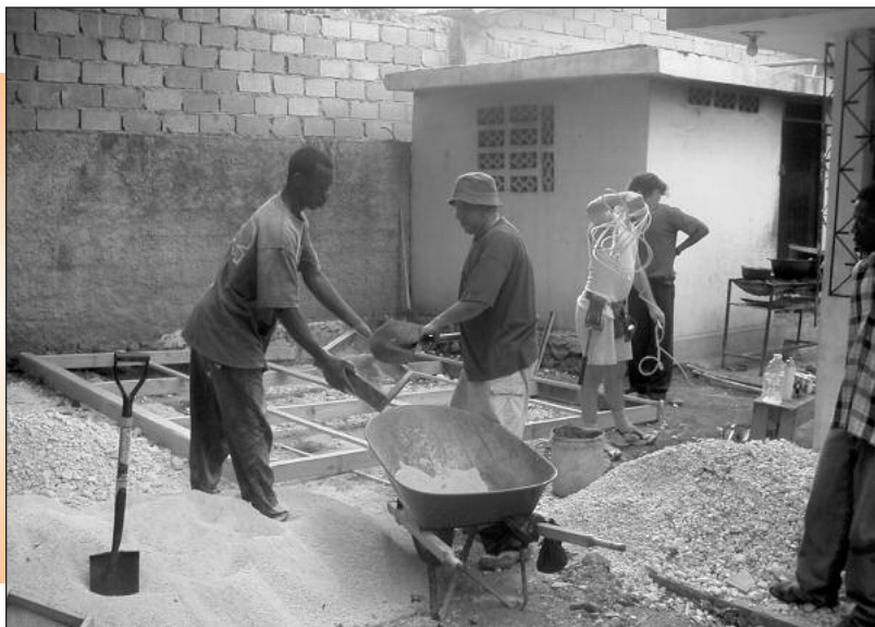
Sifting gravel for the concrete floor of the new outdoor kitchen.
