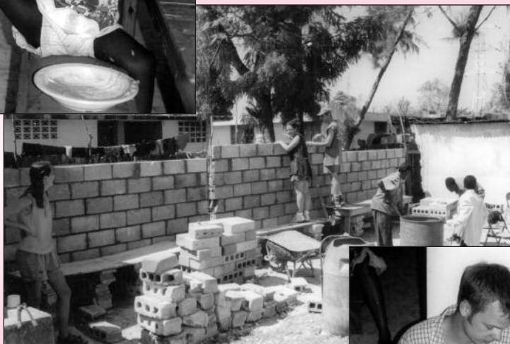
Team members building a wall at Coram Deo.
