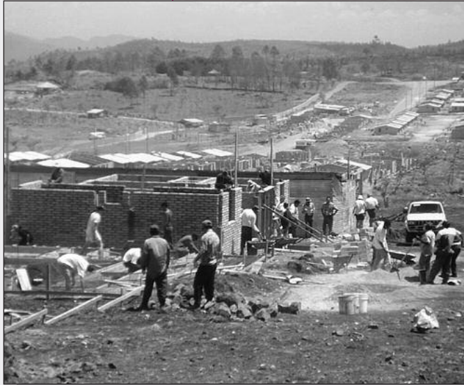
Worksite: Building in progress by the team.
