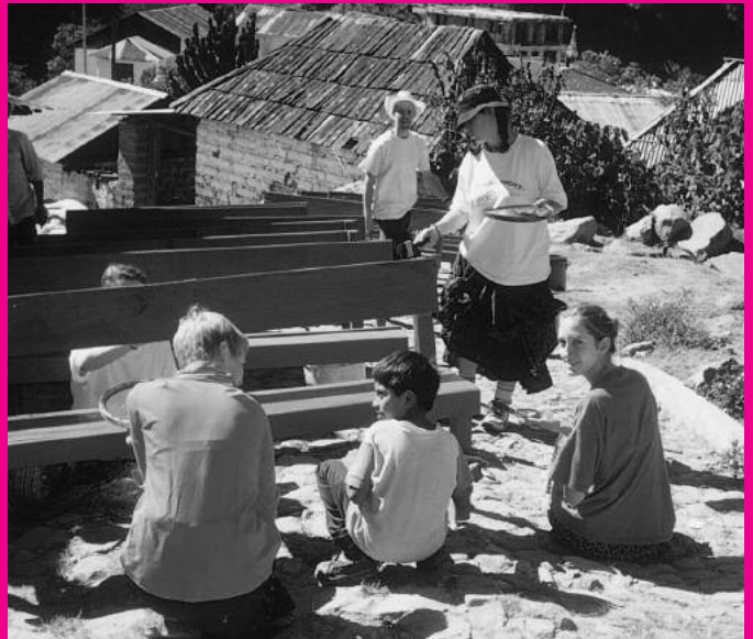
Faithworks in Guatemala – building and painting church benches.
