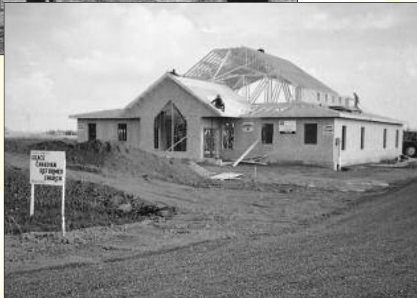
November 9, 1998. The church building is taking shape.
