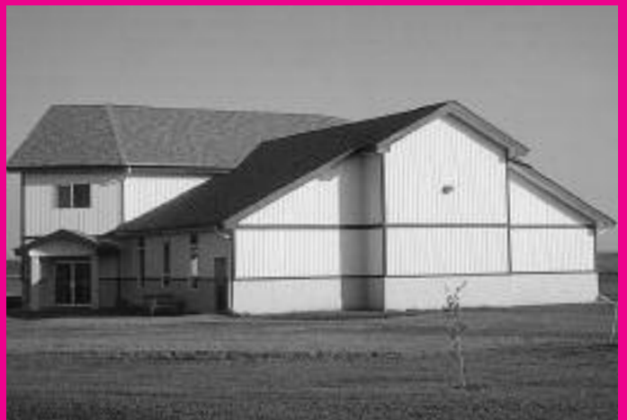
Canadian Reformed Church building at Calgary, AB
