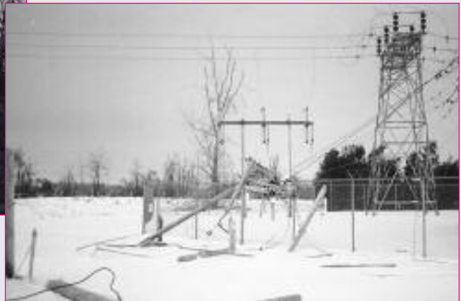
Transmission lines and power substations are ruined.
