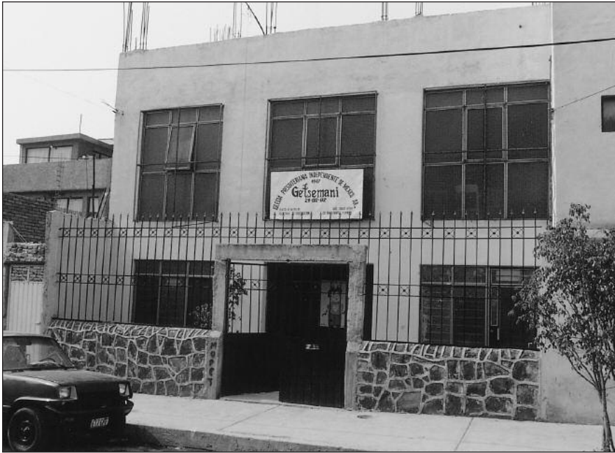
The church building of the Gethsemane IPCM. They are saving for a third and final floor. The auditorium encompasses the first two floors, with a balcony. Our group worshipped here on Sunday morning, May 11.
