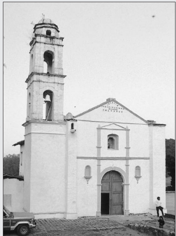
The IPCM church building in Miahuatlan, a lonely village of the Mazahua Indians, high in the mountains west of Mexico City (at an elevation of about 10,000 feet). This is a seventeenth century church building of abode, one of the very few churches that has actually changed ownership from Roman Catholic to Protestant. We worshipped here Sunday evening on May 11.
