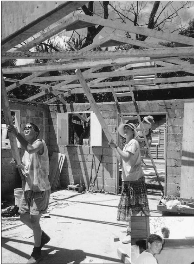
Putting up the trusses on the church.
