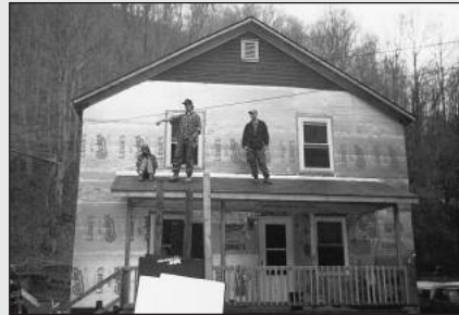
Insulating an Appalachian home
