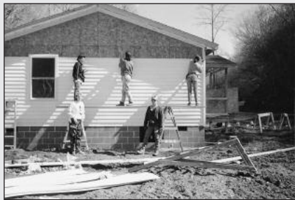
Installing siding on a new house
