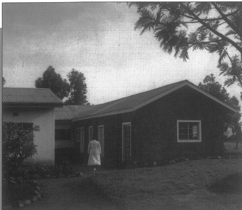
Office wing at Achego Children's Home
