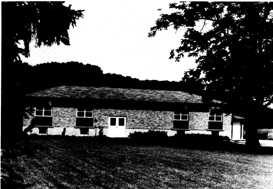
Front of school building.
