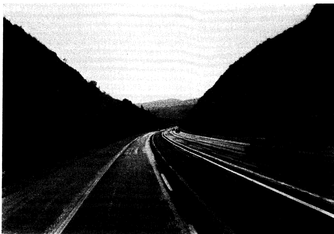
New highway to Bethel.
