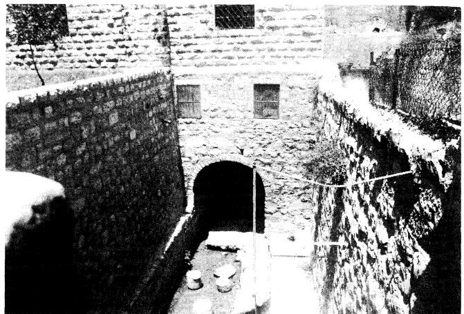
The Pool of Siloam.
