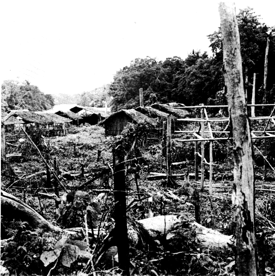
The new Heyokubun under construction.
